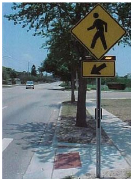
Example of Rapid Flashing Beacon on Crosswalk Sign
